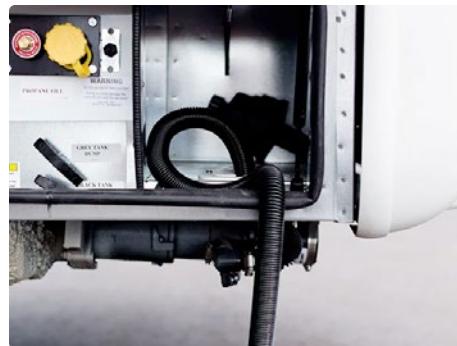
Macerator Sewage Discharge With Manual Disconnect
